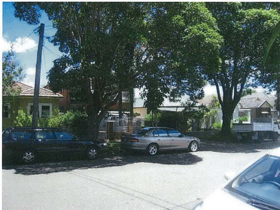
Photograph 3: 12-16 Sixth Avenue viewed from across the street
